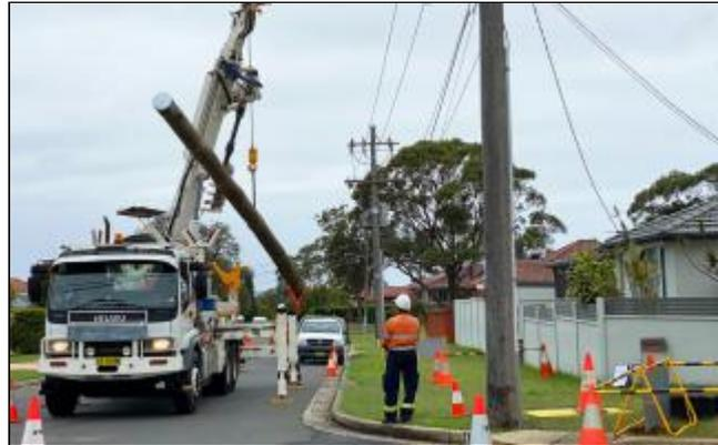
This extensive Hands-On course covers Erecting Poles And Attaching Crossarms Erecting Poles Using Earthborer And By Manual Method Facing And Aligning Poles Installing Single, Double, Sidearm, Buck, And "H "Type Crossarms and the equipment and methods that can be used to set and replace utility poles.
